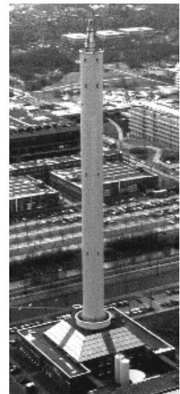
Figura 4- Torre do ZARM, Bremen.
